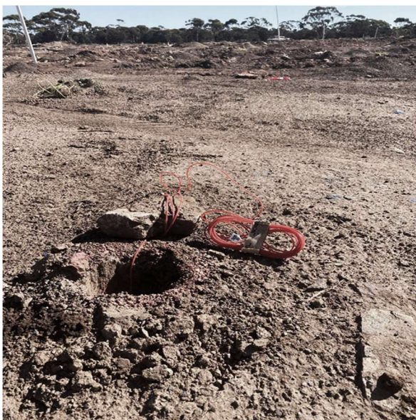
First Blasting at Jeffreys Find in May 2023
