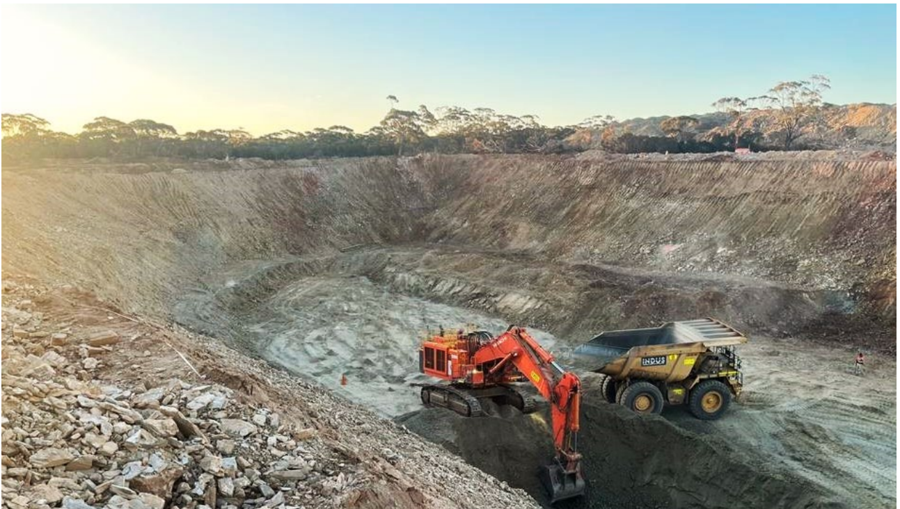
The initial pit takes shape at the Jeffreys Find Gold Mine.
