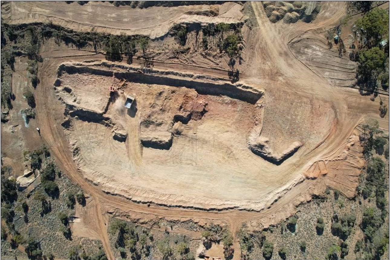
The initial pit takes shape at the Jeffreys Find Gold Mine.
